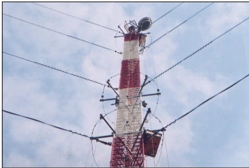
Figure 2. WHIT-FM tower, with radomes, reflectors, and STL near the top. Vertical detuning skirts are attached, allowing placement close to the AM array.
