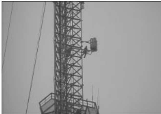
Tower technician employed by 'Reflections' of North Carolina installs antenna for WISC DTV. Photo by Leonard Charles.
