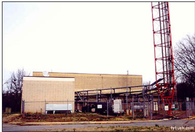
The master FM transmitter building
